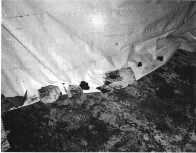
View of the barricade from the inby side.
