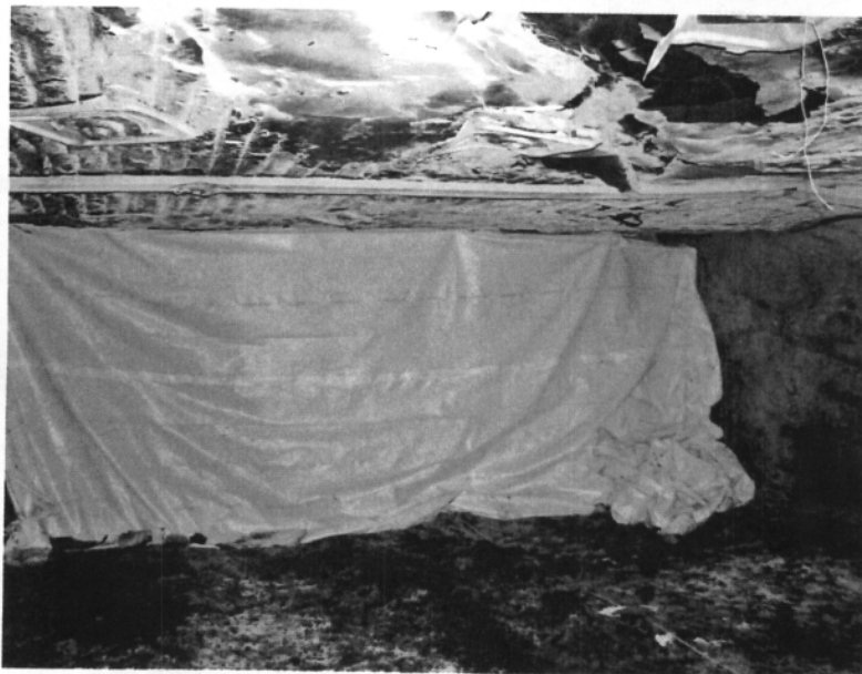
Outby view of the barricade constructed by the 2 nd Left crew in an attempt to isolate themselves from the contaminated mine atmosphere.
