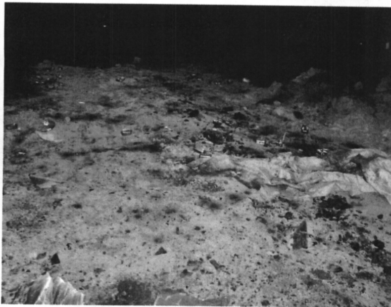
Discarded pieces of the 2 nd Left crews SCSR's were found in the #7 entry at about the eleven block. The picture indicates all the miners donned their rescuers at the same time at this location.
